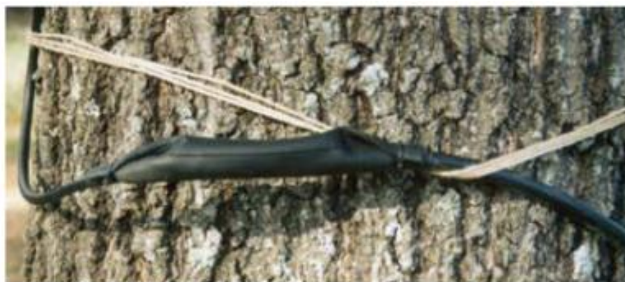
Completed coax connection waterproofing system.
